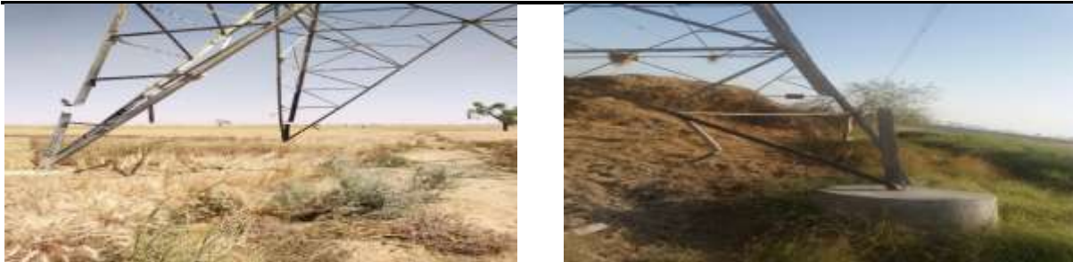
Figure 5: Impact of Sabotage in fragile locations resulting in disruption first climatic hit
